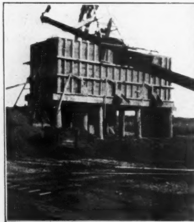
The Screening and Storage Plant
